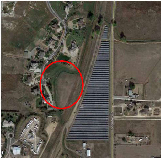
Brighton PV Solar, Adams County, CO June 2016
