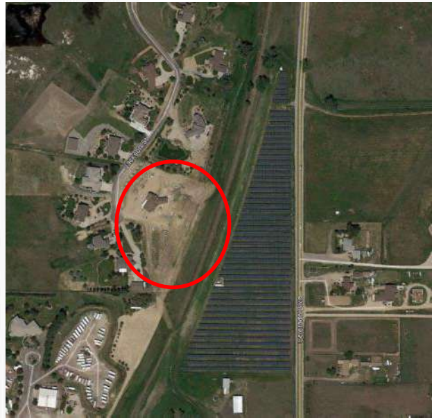
Brighton PV Solar, Adams County, CO June 2017
