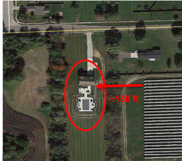
Dominion Indy III Solar Farm October 2016
