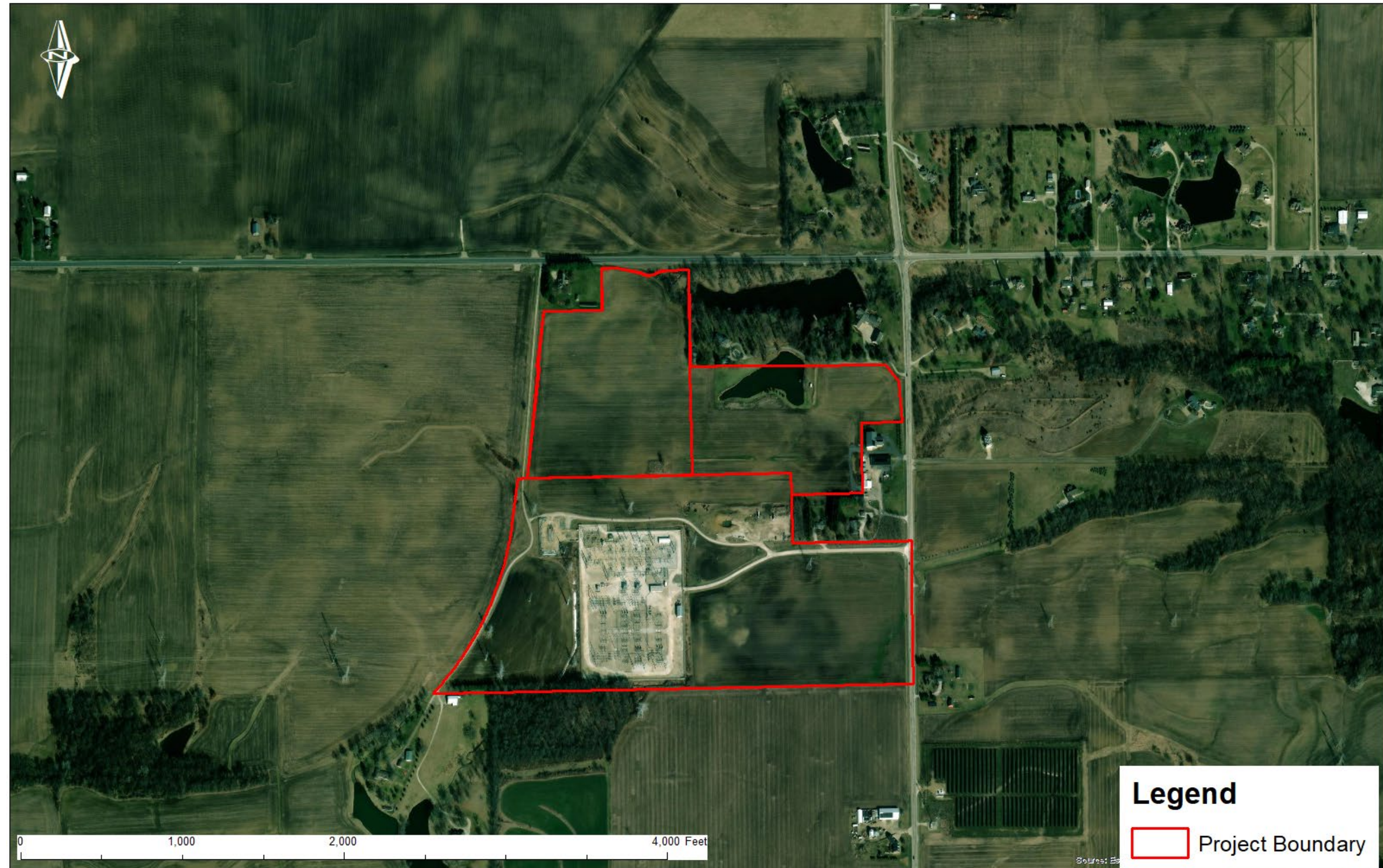
FIGURE 2. LUMINA BESS AERIAL
